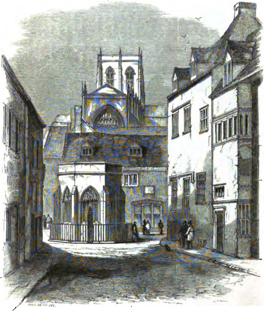
CONDUIT, EAST END OF THE CHURCH.
